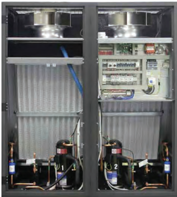
50 kW upflow 2 circuits direct expansion air conditioner
