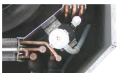
Condensate pump integrated in all sizes
